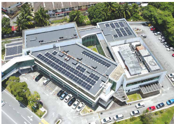
Solar Hospital Columbia Asia Seremban
